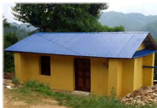
Figure 2: Completed Earthbag House in Gorkha, built by Good Earth Nepal ( Good Earth Nepal, 2015 ).
