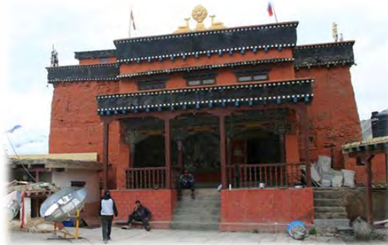
Figure 3: Kagbeni Rammed Earth Monastery, Nepal, built 1429 (Geiger, O., 2013).
