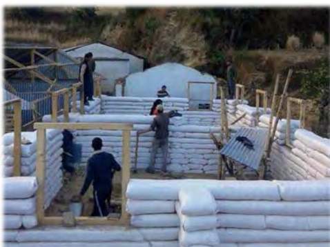
Figure 1: Earthbag Construction in Makwanpur, built by Good Earth Nepal ( Good Earth Nepal, 2015 ).
