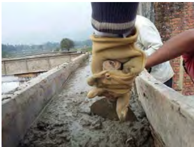
Figure 16: Concrete Bond Beam (Good Earth Nepal, 2015)
