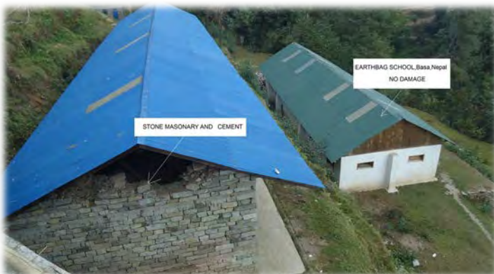
Figure 10: Earthbag School in Basa, Nepal built by Small World next to a damaged stone building (Good Earth Nepal, 2015)
